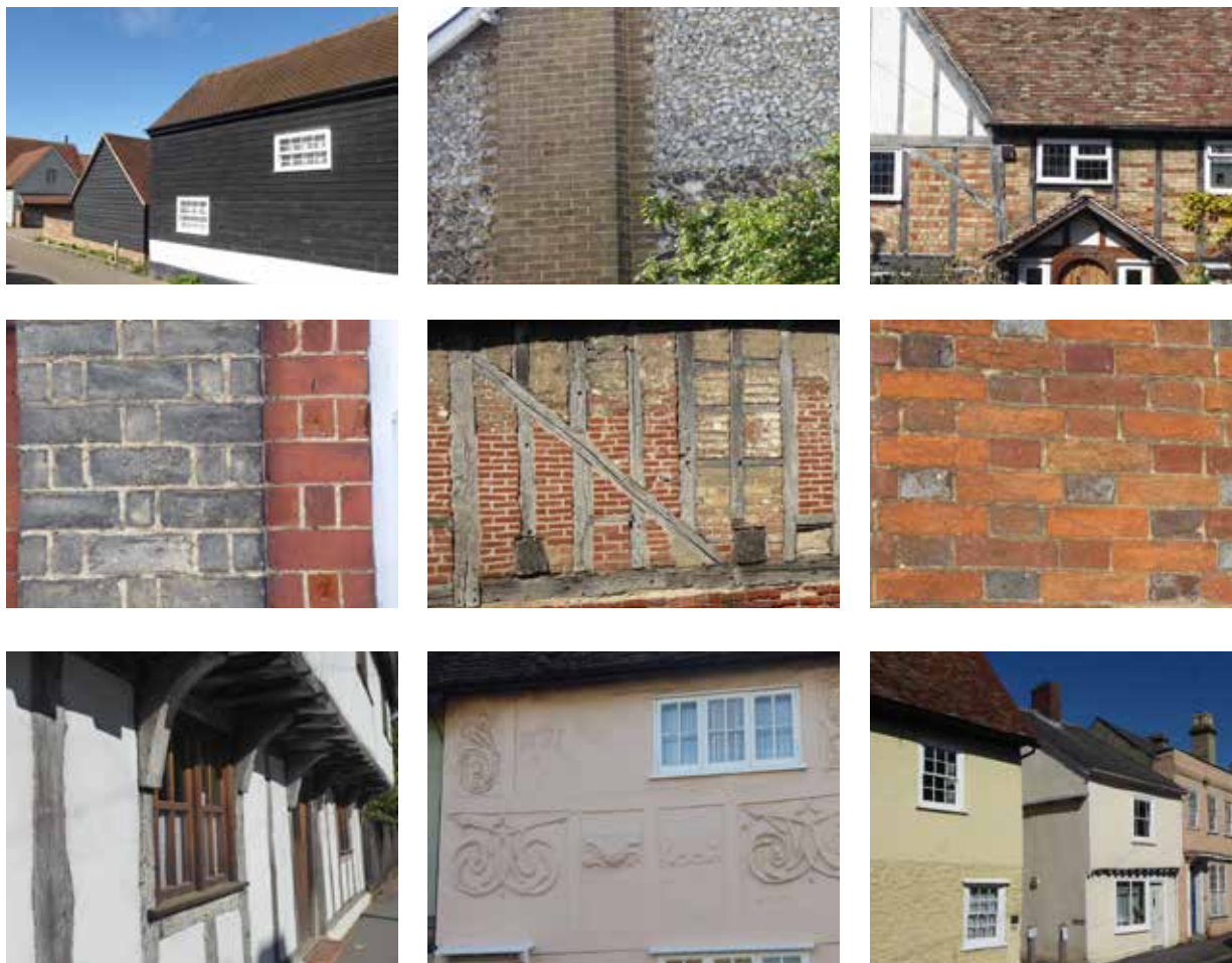
Figure 33: Examples of different wall materials within the Character Area. Clockwise from top left: Weatherboarding, Flint and Brick, Timber framing with sections of brick nogging and render infill, Flemish bond brickwork, Rendered and jettied houses, Pargetting, Exposed beams with render, Rat trap grey brick, Exposed timber with nogging
